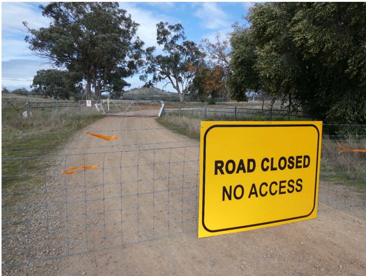
Caption: Permanent stock fencing installed closing off existing access with reflective sign.
