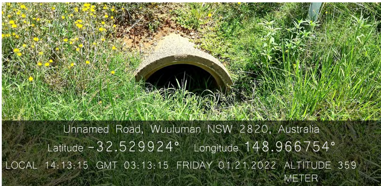
Photograph 4.2 Existing culvert crossing at Watercourse A
