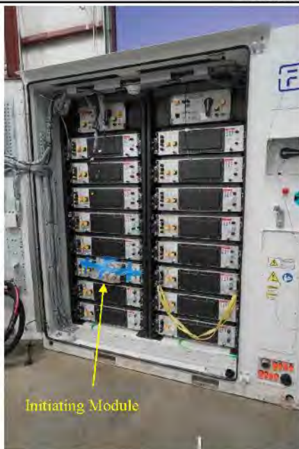
Figure 3: A photograph of the initiating module installed in the initiating unit.
