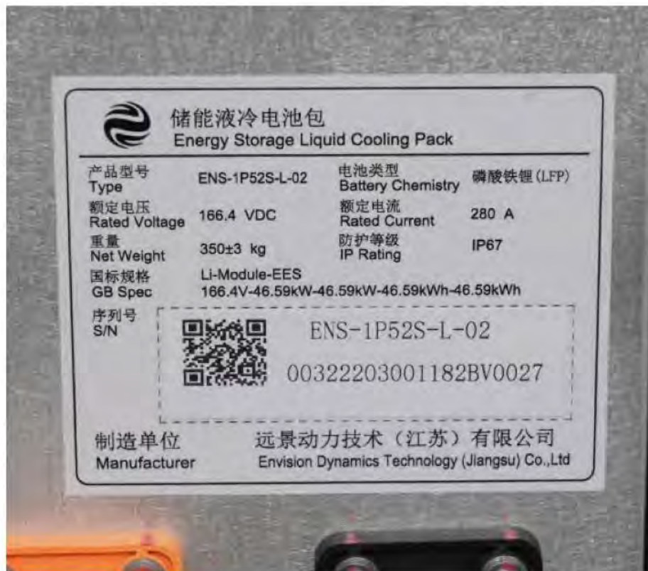
Figure 6. AESC BDBT initiating module nameplate.
