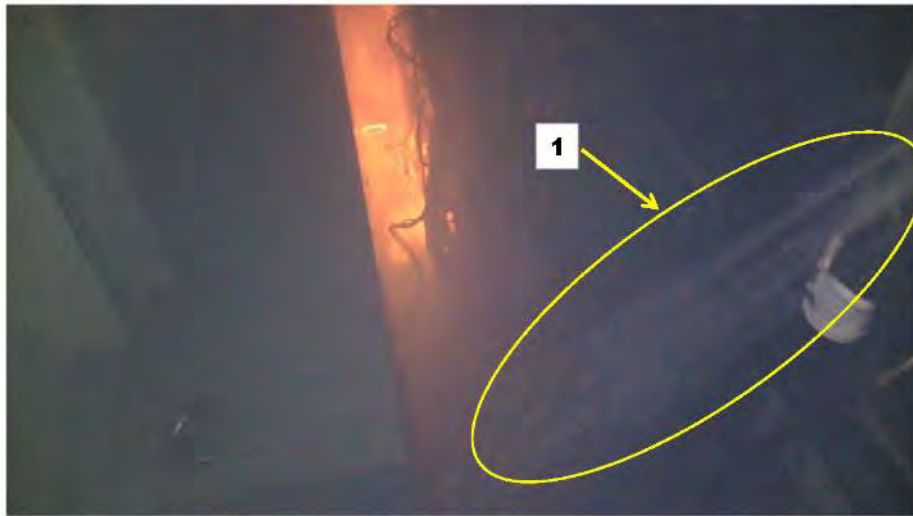
Figure 19. A screen capture shows coolant lines leaking inside the initiating unit while flames are also visible (1:53).
